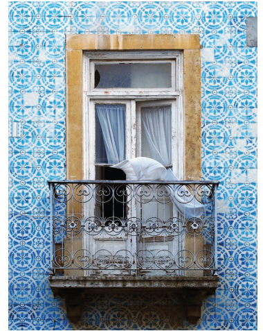
Image 2 Many buildings in Portugal are covered in azulejos with a simple, repeating geometric design.
