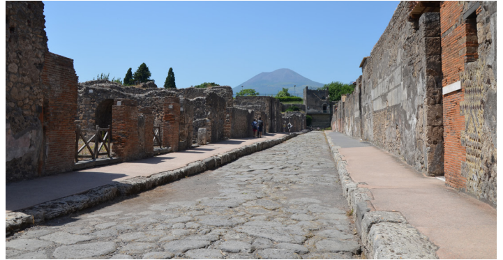
Large stone blocks, curbs, and pedestrian walkways were all part of ancient Roman road design.
